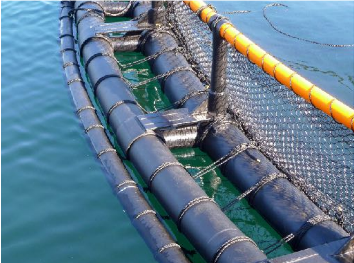
35m-diameter cage with balanced stanchions, 355/315mm floating pipes, Kikkonet. Oita, Kyushu, Japan
